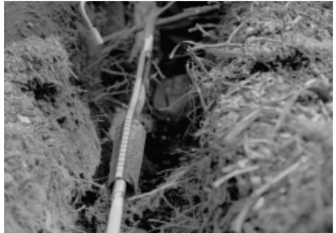
The CWST sleeve is simply wrapped around the damaged cable area and shrunk with a standard jointer's torch.
