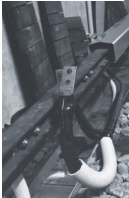
Photos: Electrical failures frequently result when birds perched on catenary wires make contact with the bridge as they fly away to avoid oncoming trains. This problem is overcome by insulating the catenary wires with Raychem FCSM tubing as shown here.
